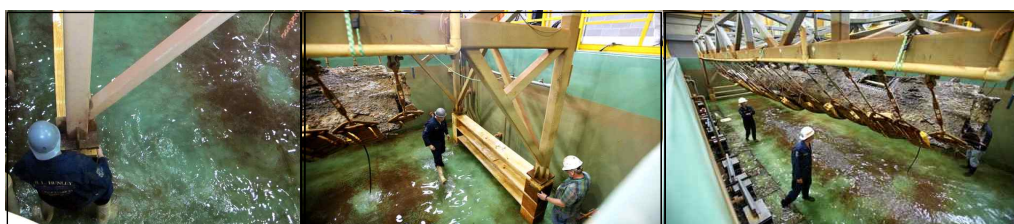
c) & d) A worker positions a wooden platform beneath the truss.
