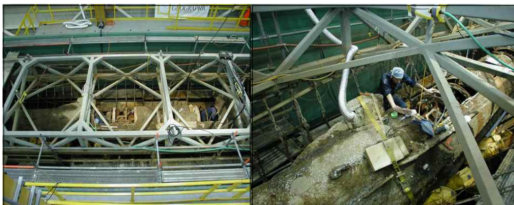
m) General view during the central compartment excavation. n) Excavation of the front area.
