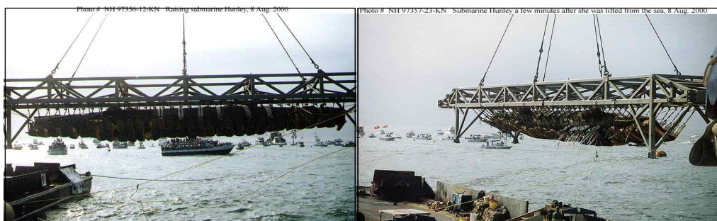
a) Suspended from its supporting truss (USN). b) Being placed on the barge (USN).
