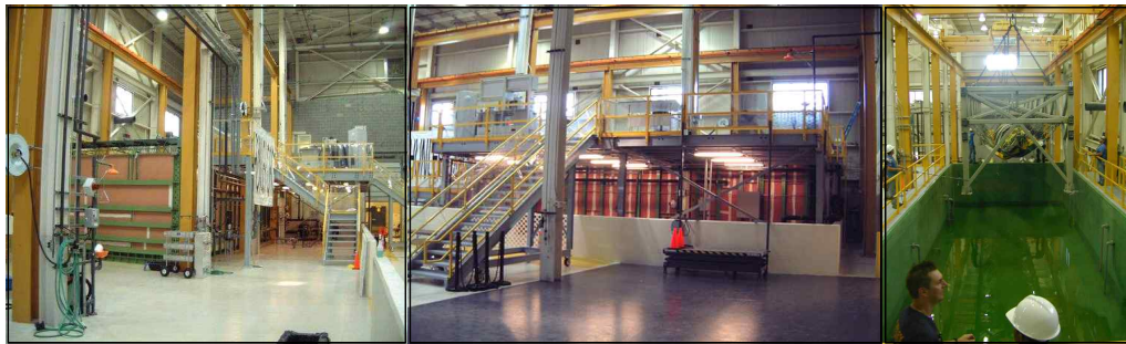
b) The outside of the treatment/storage tank. c) Exterior view of the tank and the tank area. d) View from the bottom of the tank.
