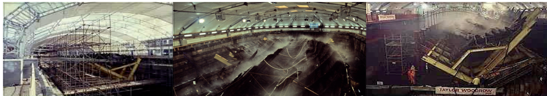
d) Building the ship hall. e) Mary Rose being sprayed with water. f) Turning the ship.
