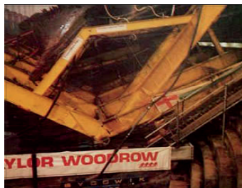
g) During the sliding operation.
