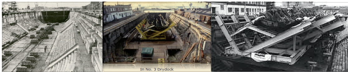
a) No.3 Drydock ready to receive the hull. b) & c) In No.3 Dry dock.
